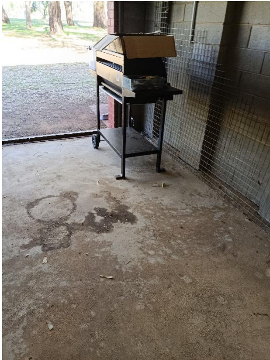
Floor Before Cleaning
