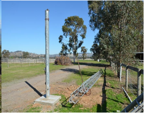
Alan's current Project, the new tower
