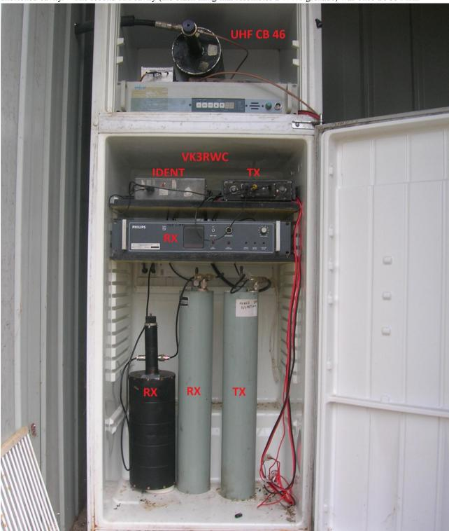
analogue mobile phone tower ¾wave cavity filter. The plunger had been shortened to work as a ¼wave filter for 477 MHz. The plunger has been inverted, lengthened, and made into a tubular piston trimer capacitor (using a piece of LDF 550) to resonate it at 2 metres. The thing that really surprised me was, that I could get a higher Q notch with it, than I could with the full sized 3 inch cavity.
