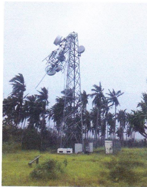
A mobile phone and communications tower located in Vanuatu, damaged by one of this years cyclones. Image by: dailypost.vu
